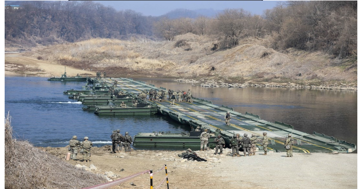
U.S. and South Korean soldiers build a joint bridge during a wet gap crossing exercise in South Korea, March 14, 2024 .
